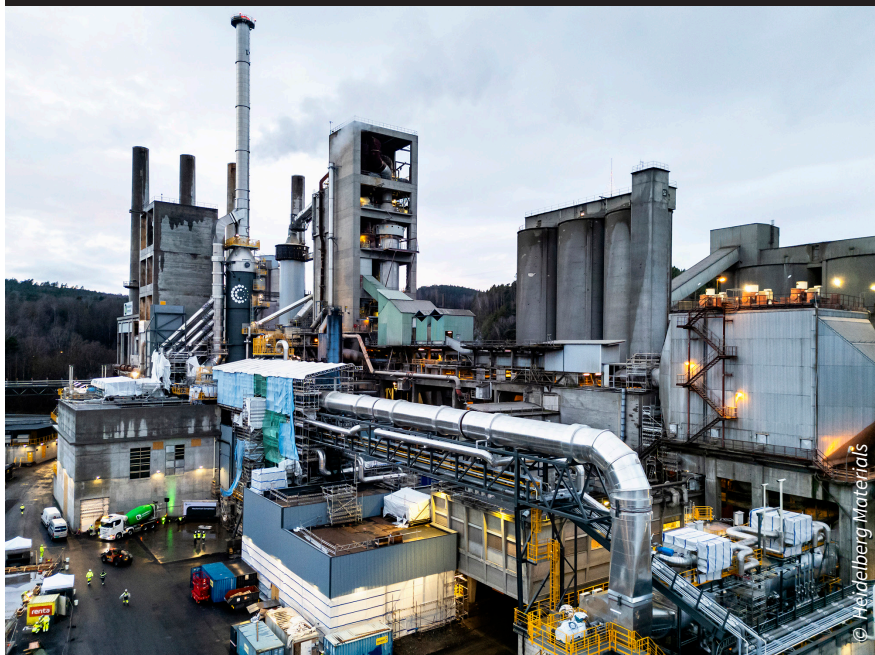
In June 2025 Heidelberg Materials inaugurated Brevik CCS in Norway, the world's first industrial-scale carbon capture facility in the cement industry
